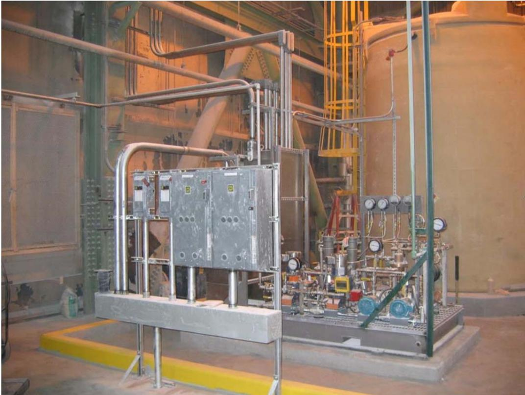
Figure 5. ADA<sup>®</sup> RESPond™ Injection Equipment: control skid and chemical storage tank.
