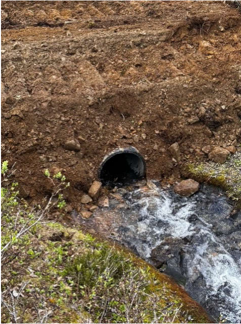
Plate 019: Final installation of temporary crossing at KN003.
