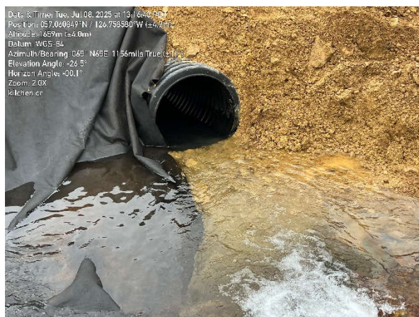
Plate 008: Photo KW009. Full barrier, 10m falls, full barrier to Plate 008. Geofabric installation at inflow of 900mm culvert at site KN001. upstream fish passage at FBZ, approximately 500m upstream of Amazay Lake.
