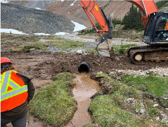
Plate 009: Culvert 1 at site KN002.
