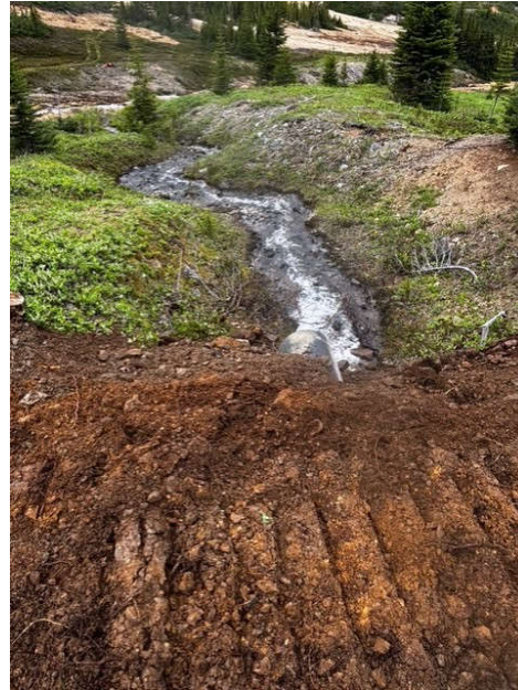
Plate 020: Final installation of temporary crossing at KN003.
