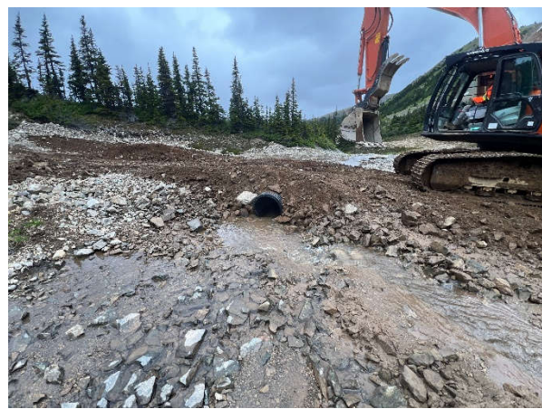
Plate 014: Culvert 2 inflow at crossing site KN002 with riprap armouring placement.
