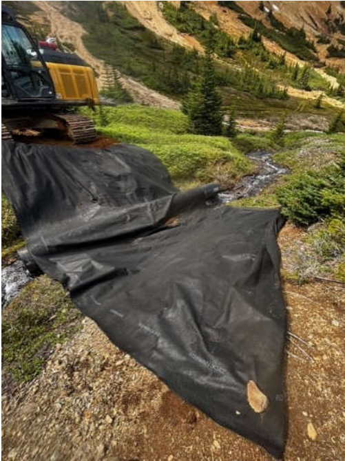
Plate 017: Installation of geofabric at temporary crossing KN003.
