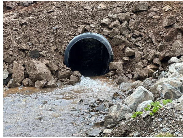
Plate 012: Culvert 2 inflow at crossing site KN002 with riprap armouring placement.
