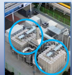
Two modules are used for a 2.8MW power plant
