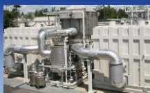
2.35 MW SureSource Hydrogen™ 2.35 MW Power plus 1270 kg/day Hydrogen
