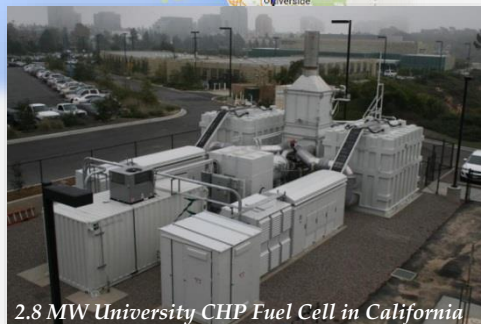
2.8 MW University CHP Fuel Cell in California
