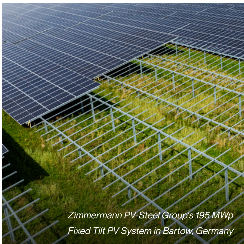
Nextpower power conversion technology with modular, flexible system architecture and serviceability
