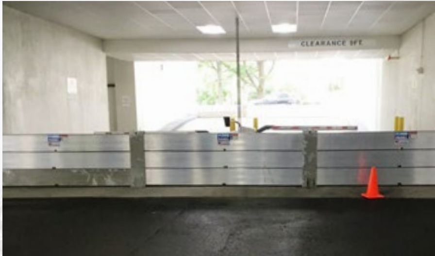
Two Commercial Place, Norfolk, VA – OPI Flood panel barriers
