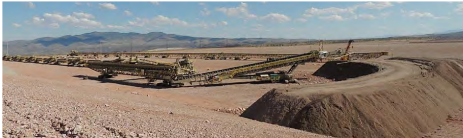
Figure 14.5: Example Stacking System Operation (Terra Nova Technologies)
