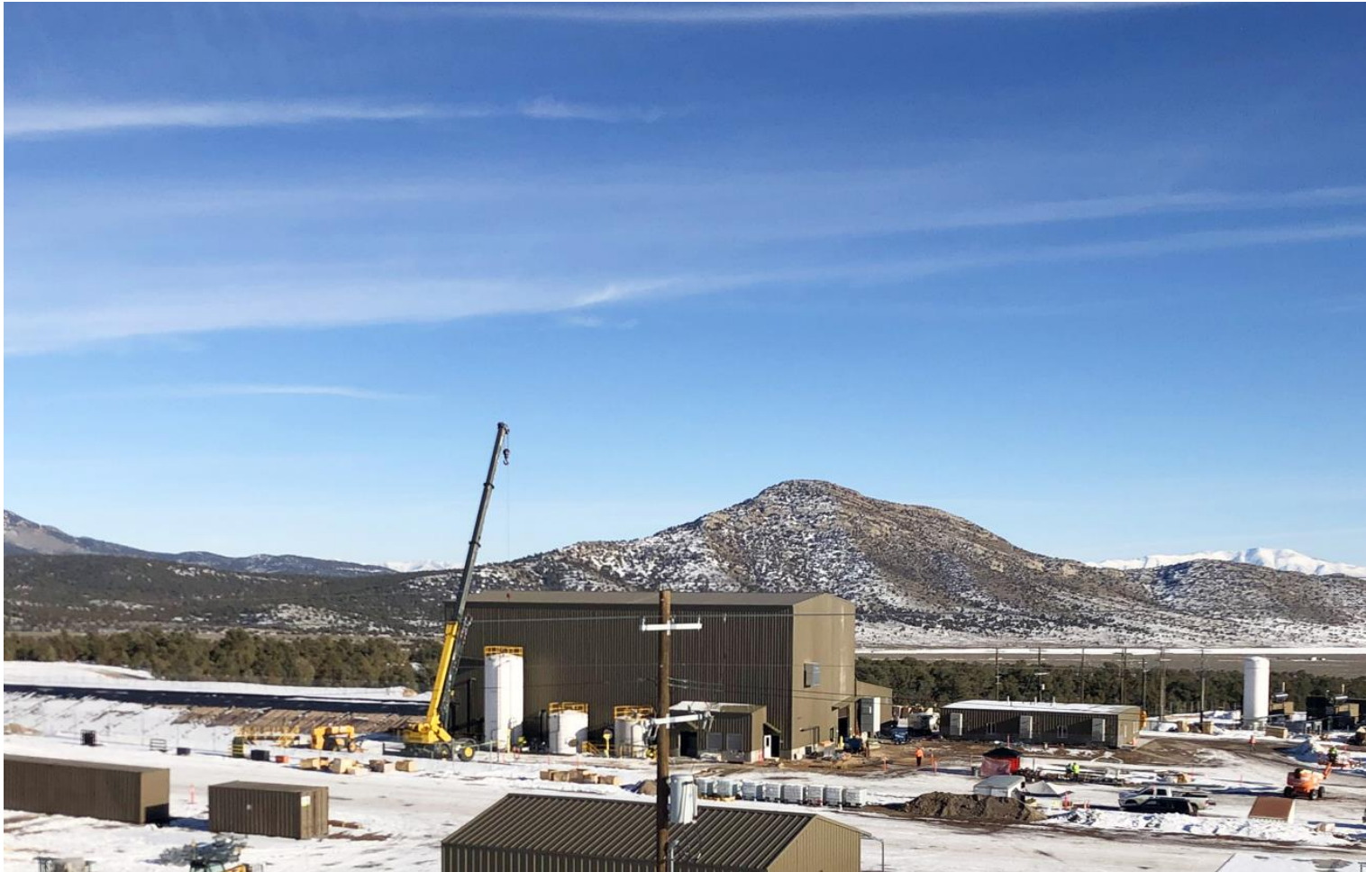
Gold Process Plant Building Complete
