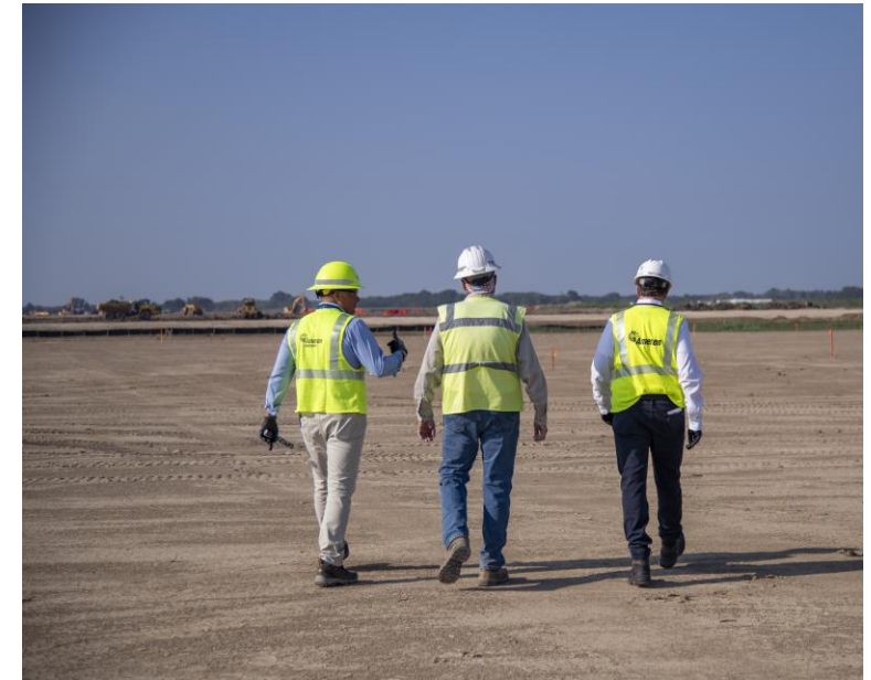
Construction began Q2 2026 on both Amazon and Google data center sites located in Montgomery County, MO.
