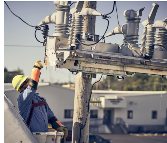
A lineman inspects an intellirupter, a smart switch, that can automatically reroute power until a line is fixed, improving reliability by up to ~50% more than a standard circuit.
