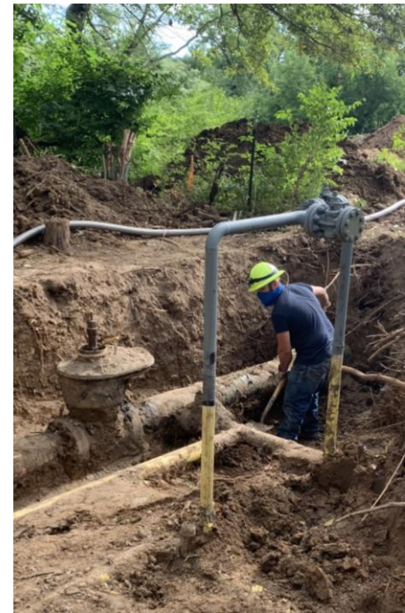
An Ameren Missouri co-worker replaces a pressure regulator station in Jefferson City, Missouri
