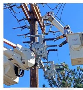
Warren County - Installation of a "Viper Switch" which will rapidly detect and isolate damage, rerouting power where possible to reduce outages and speed power restoration sometimes from hours to seconds.
