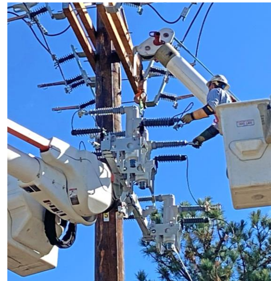
Warren County - Installation of a "Viper Switch" which will rapidly detect and isolate damage, rerouting power where possible to reduce outages and speed power restoration sometimes from hours to seconds.
