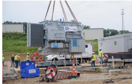
In Franklin County, crews installed a new, made in Missouri substation transformer to support reliability for over 2,700 homes and businesses.
