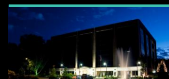
Headquarters Ground Software
