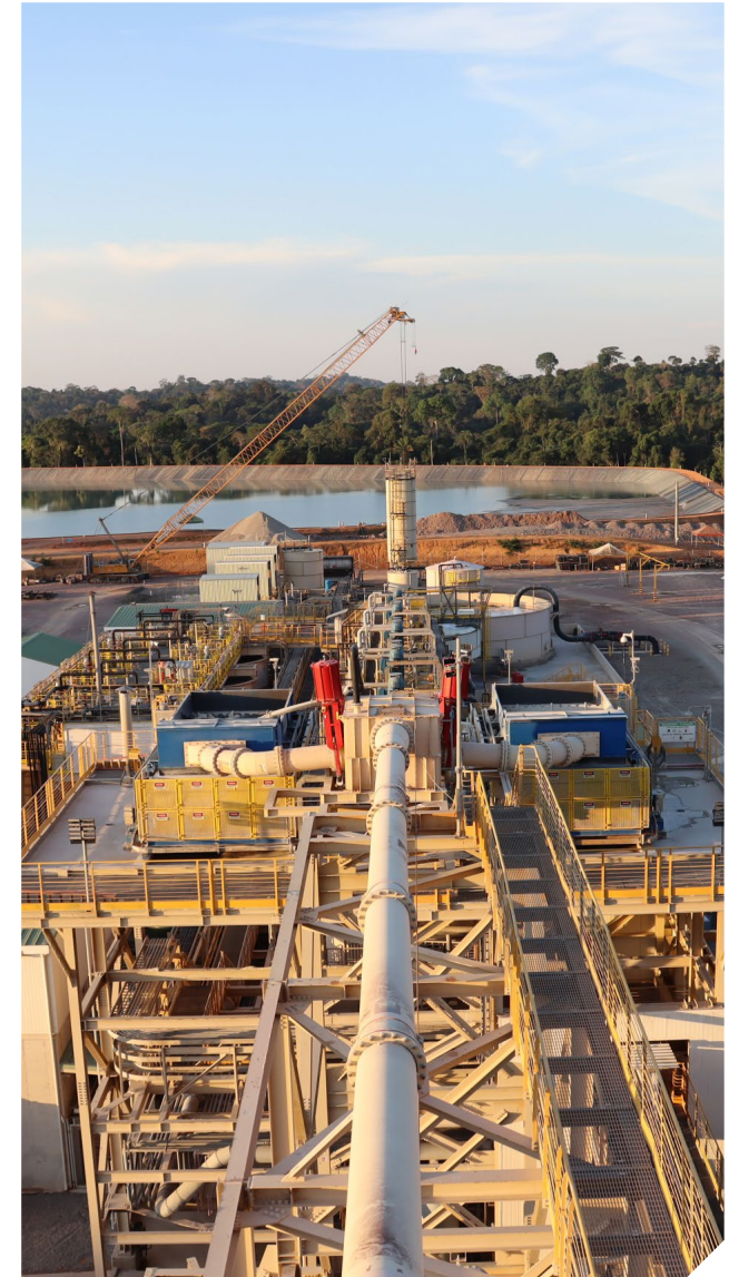
TZ Mine processing plant
