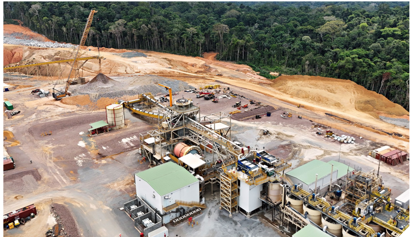
Processing Plant at TZ Mine
