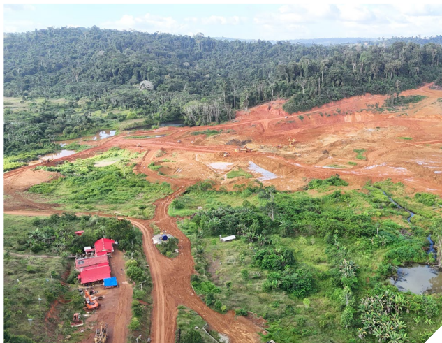
Construction of Oko West TSF
