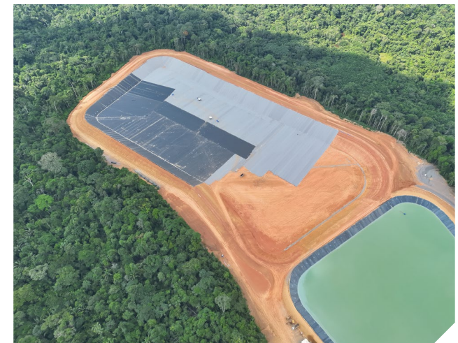
Barragem Célula 2 (CTS2) under construction at TZ Mine
