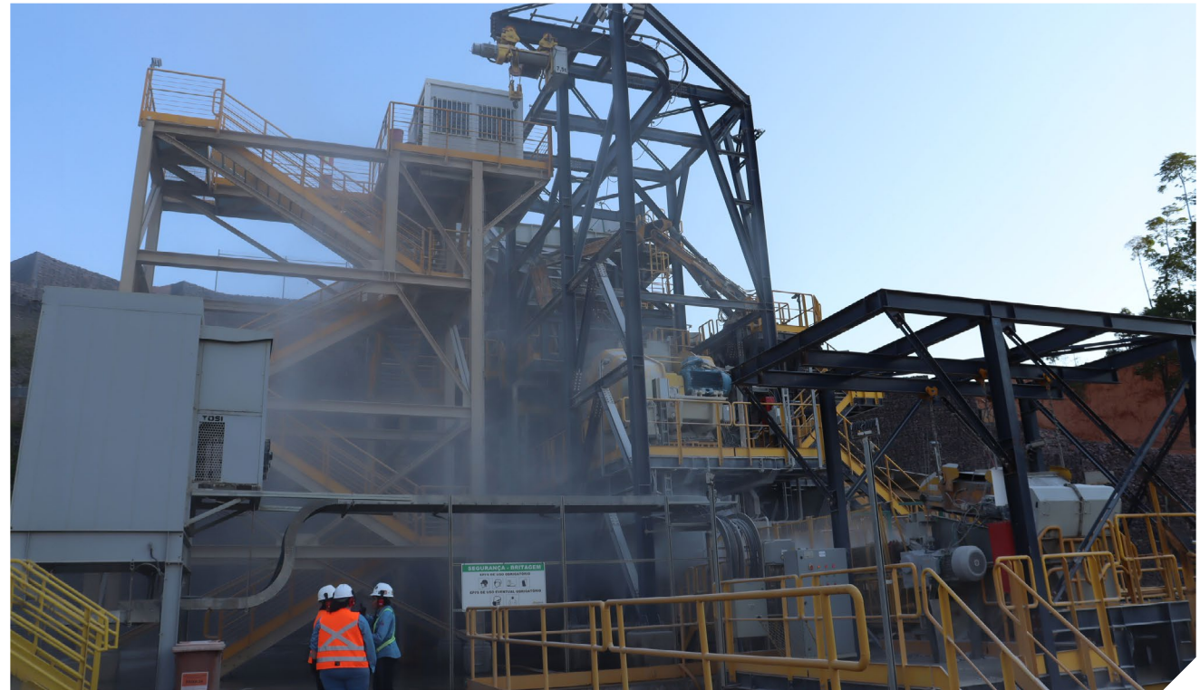
TZ Mine Processing Plant
