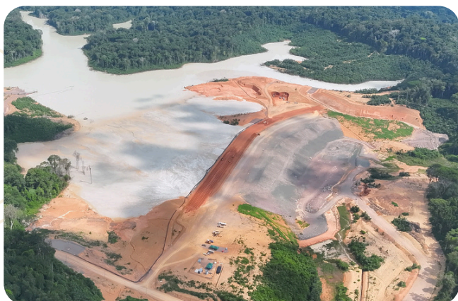
Flotation Tailings Storage Facility (FTSF) at TZ Mine
