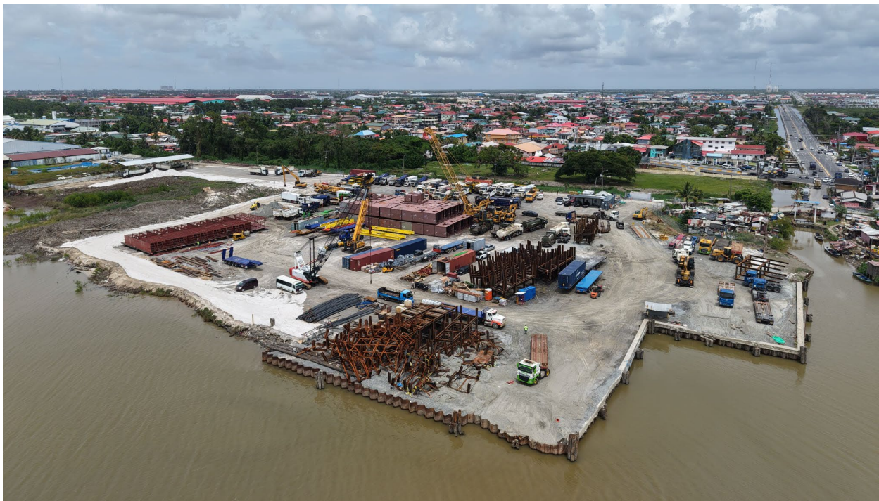
Photo: The Eccles Port Facility, located on the Demerara River near Georgetown, is currently being used to load barges destined for the Project's barge facility on the Cuyuni River.
