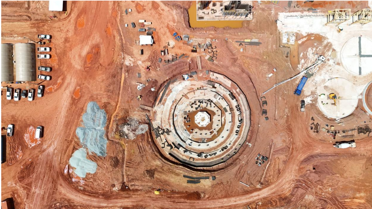
Construction of exterior rings two and three on our pre-leach thickener are more than halfway complete while ring four is being prepared to be poured in August. This work is in tandem with the associated piers.
