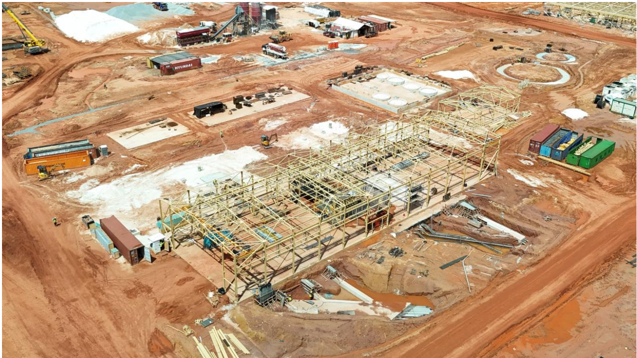
The power plant continues to advance with over 1,350 m 3 of concrete poured to date and the structural steel framing for the engine hall complete. Day tank and stack foundations are also complete while cable tray and electrical are currently being installed. Fuel treatment building (right) has completed framing.
