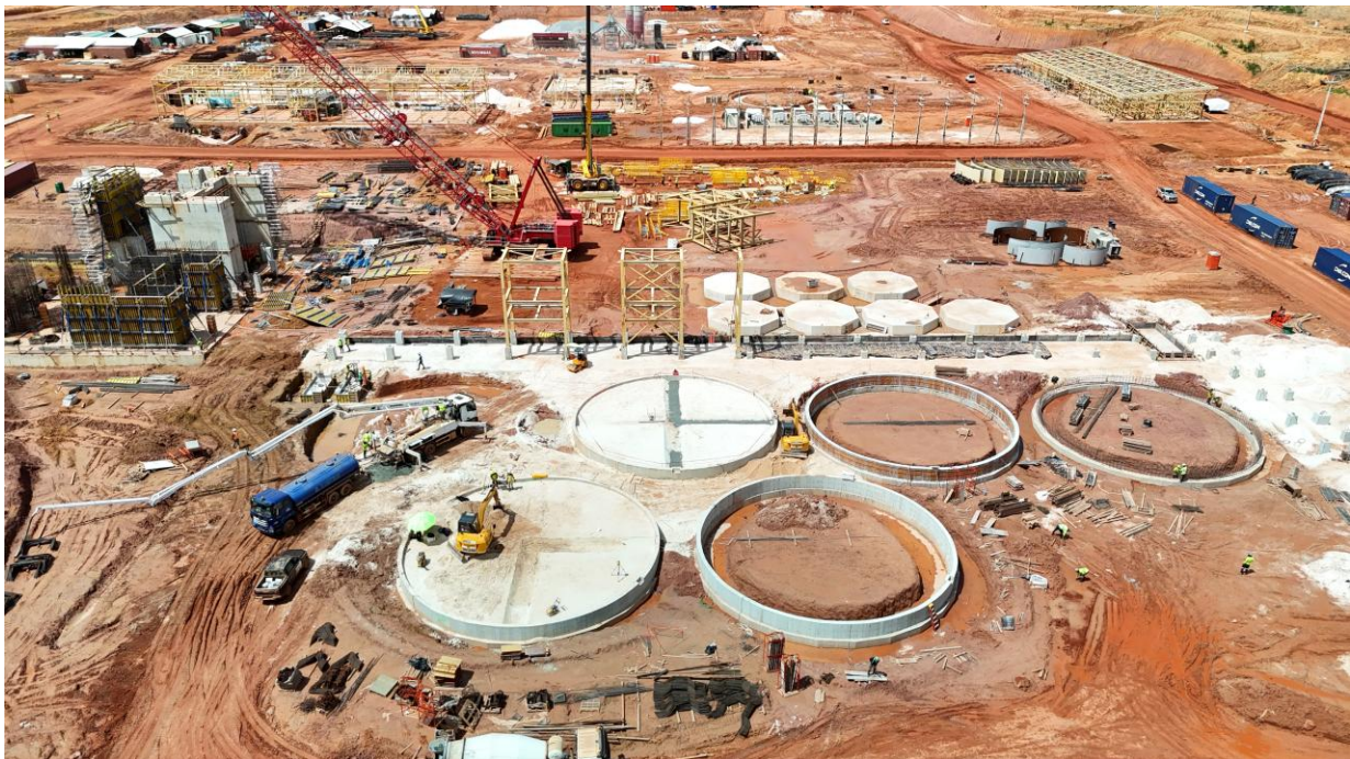
Excavation has been completed for five CIL tanks, with construction of two inner rings advancing. Foundations for all seven CIP tanks have been completed, with tank installation scheduled to commence in August. The photo also shows the commencement of the pipe rack structure.
