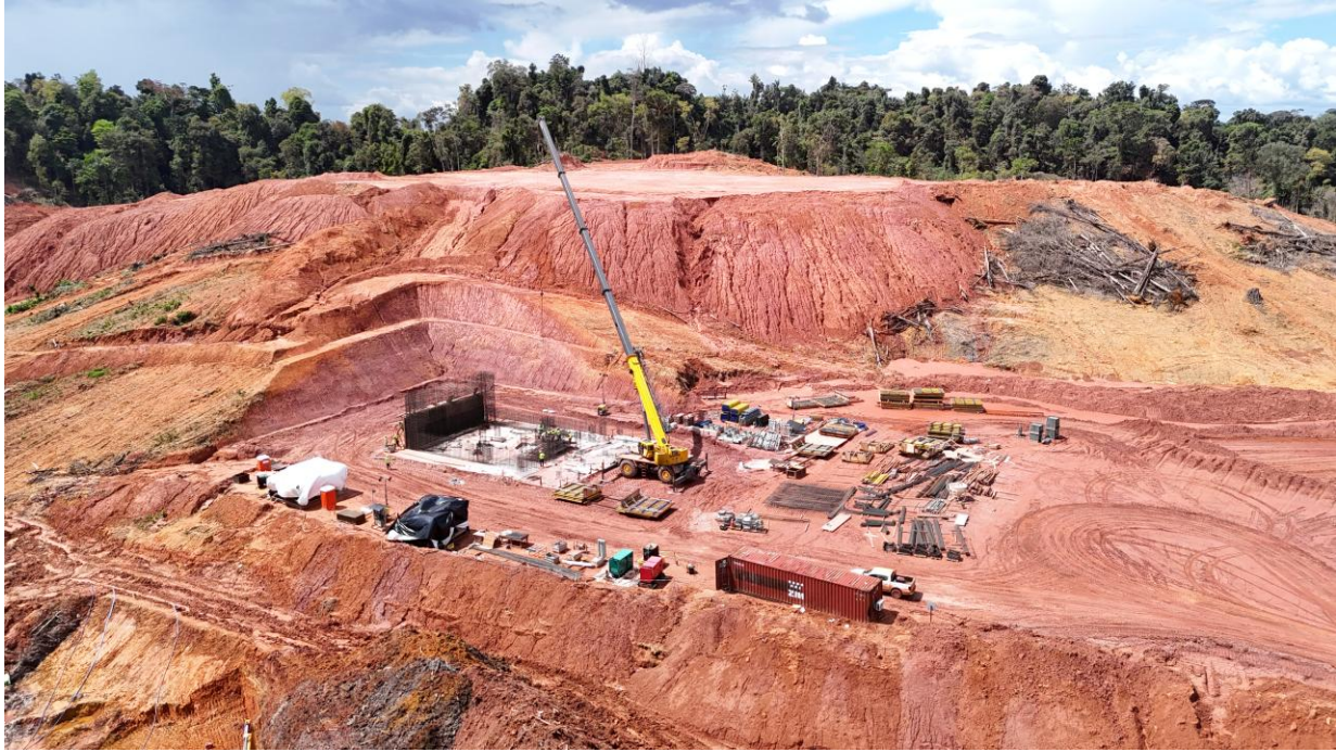
The primary crusher has advanced significantly with the mat foundation concrete pour completed. The rebar and concrete pours of the first level will commence in August.
