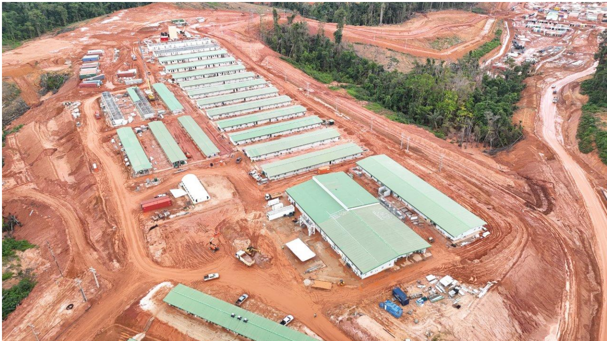
The permanent camp has over 1,400 beds, with the welcome centre, kitchen & dining hall all operational and open to employees.
