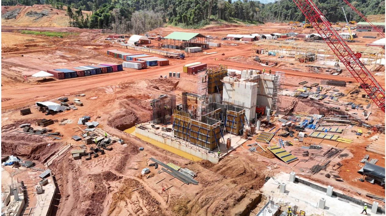
The SAG mill foundation is completed with anchor bolts and embedded plates. The first concrete pour for the ball mill foundation will take place in August.
