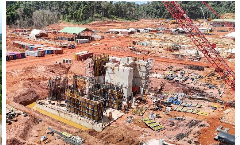
SAG & Ball Mills Progress
