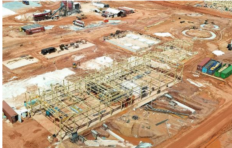
Power Plant Engine Hall Progress
