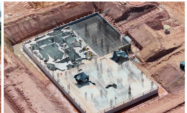
Process Plant Mill Foundation
