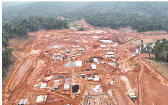
Mine Infrastructure Progress
