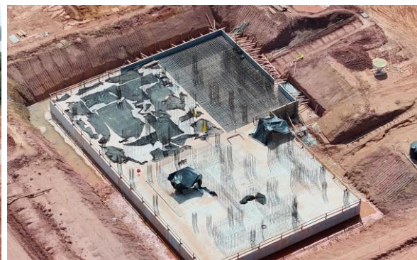
Process Plant Mill Foundation
