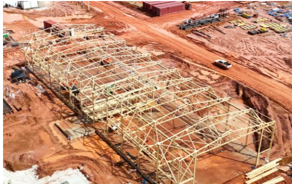
Power Plant Engine Hall Progress
