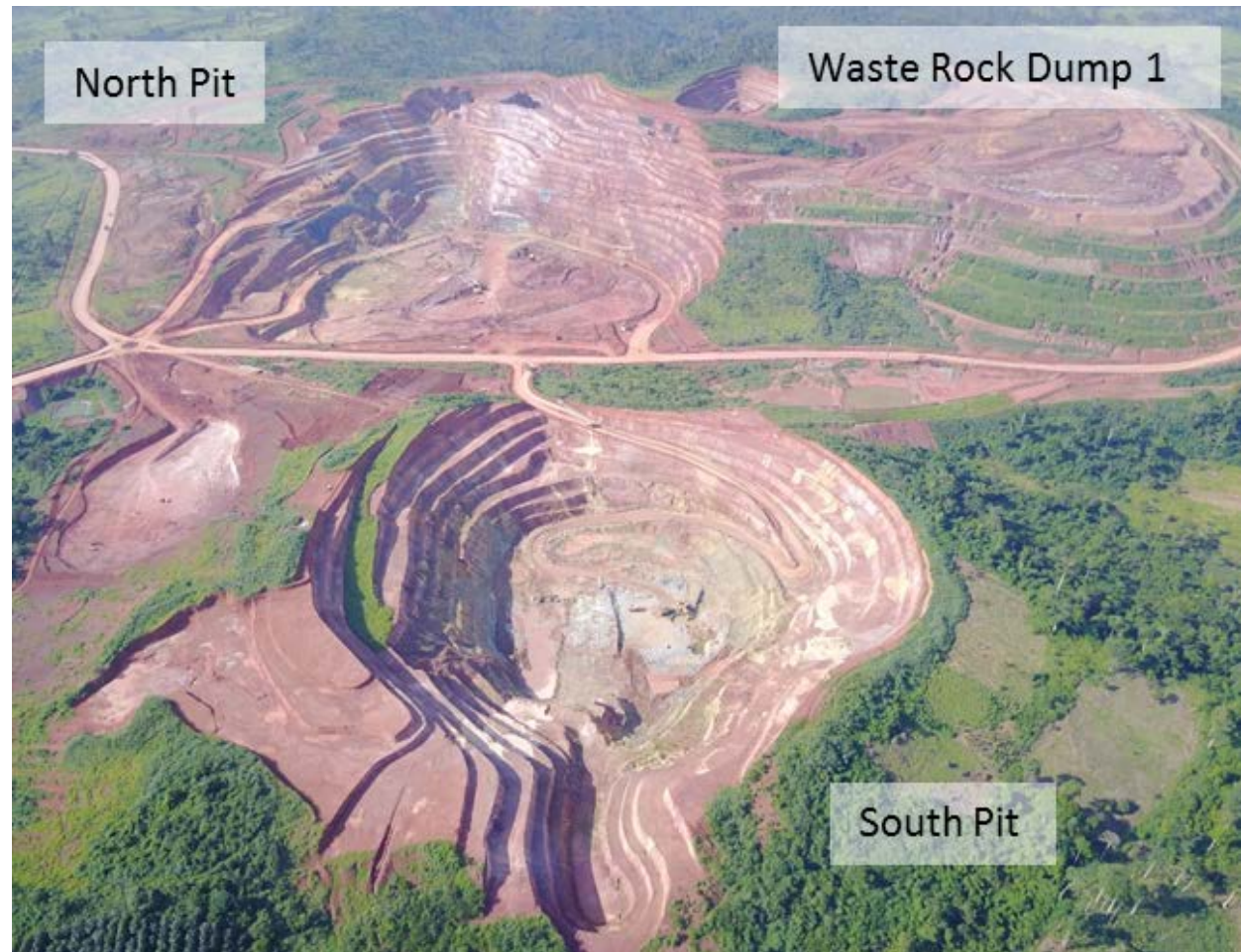
North and South pits
