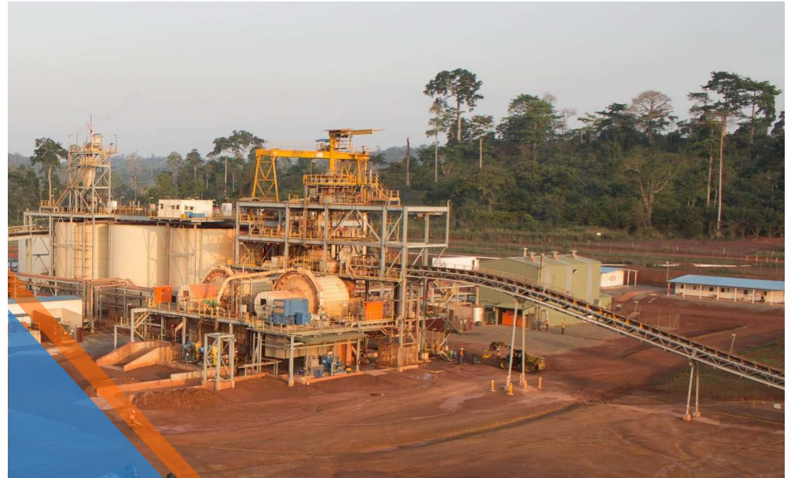
Agbaou Process Plant
