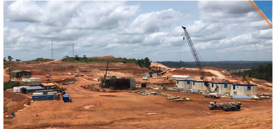
Ity Construction Site
