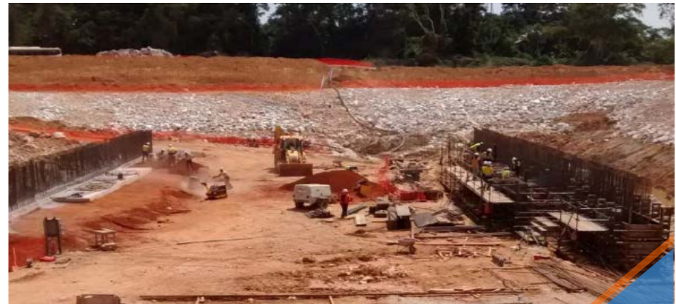
Haul Bridge Works
