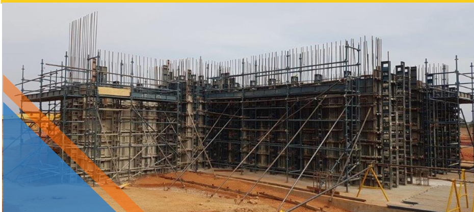
SAG Mill First Lift Poured
